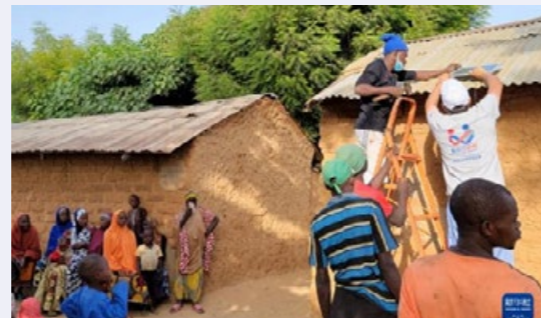
Installation of Solar Lights
