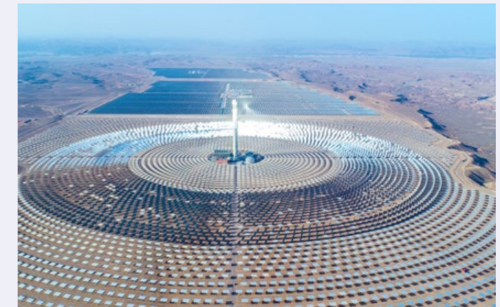
Morocco Noor III Solar-Thermal Power Station
