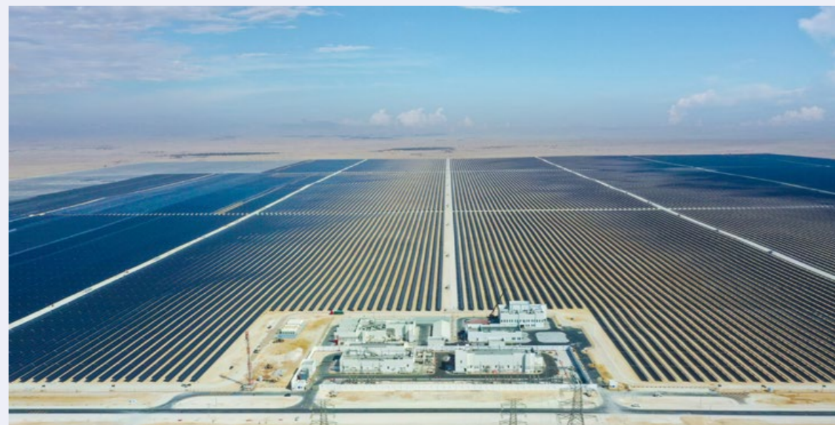
Qatar Al Kharsaah Solar Power Station
