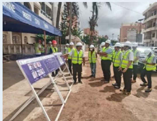
Work on site by inspection team
