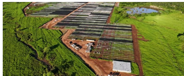
Mauriti PV DOBT Project, Brazil
