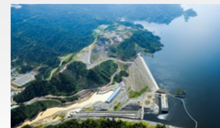
Bakun Hydroelectric Project, Malaysia
