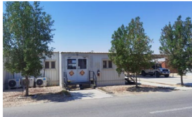
Clinic for the King Abdullah Port in Saudi Arabia: exterior
