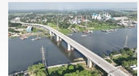
3rd Shitalakhya Bridge Project, Bangladesh
