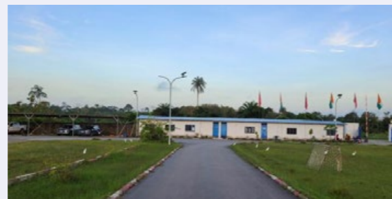
The solar street lighting system on the project site
