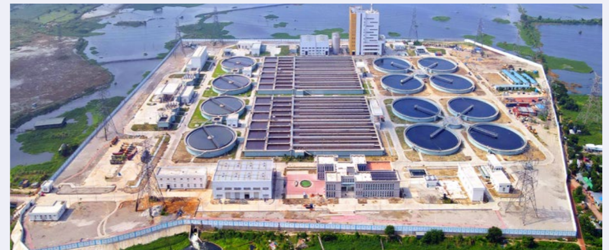
Dasherbandi Sewage Treatment Plant in Bangladesh
